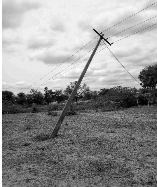
Figure 2: Electrical pole in a field leaning dangerously.
